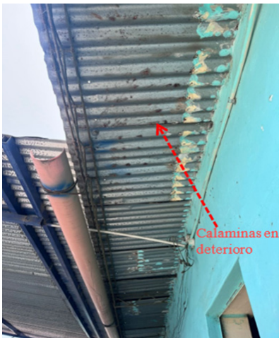
Figure 11. Detailed view of the roof in the classroom of Felix Montenegro, 5th grade Note: the figure shows the deteriorated condition of the corrugated iron roof
